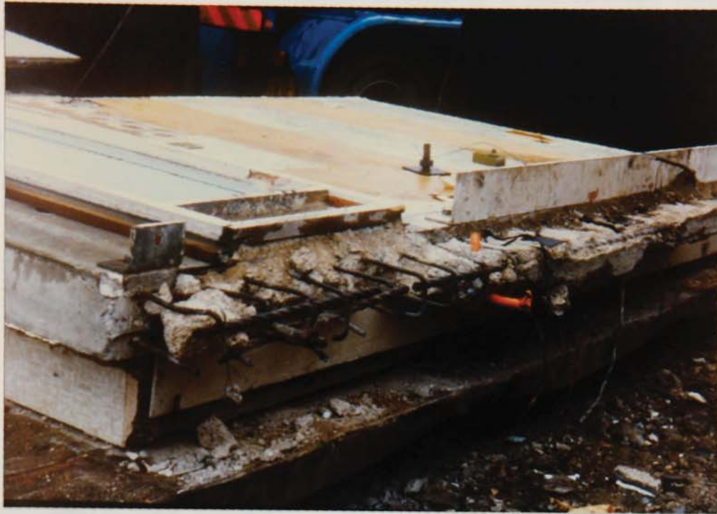
Plate 9-1 The dismantled flank walls of Ronan Point
