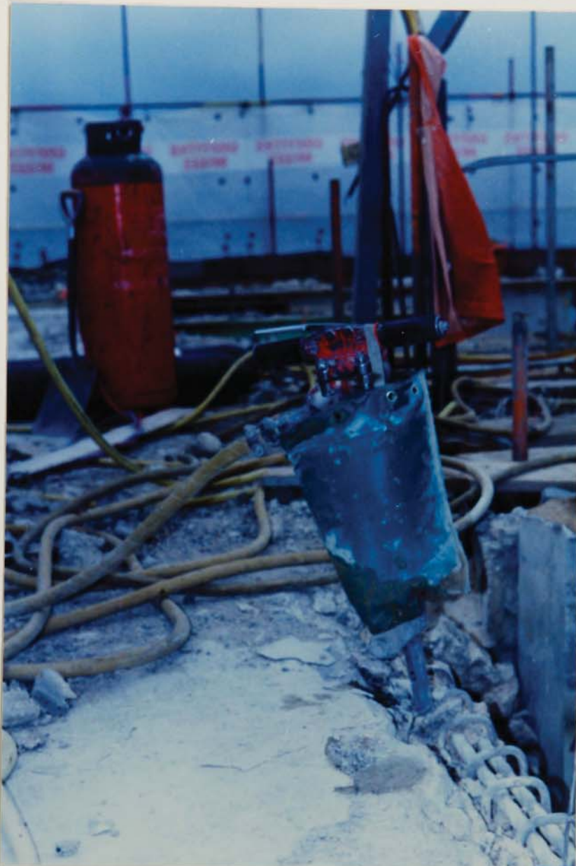
Plate X-1 The joints breaker used electrically driven compressor.
